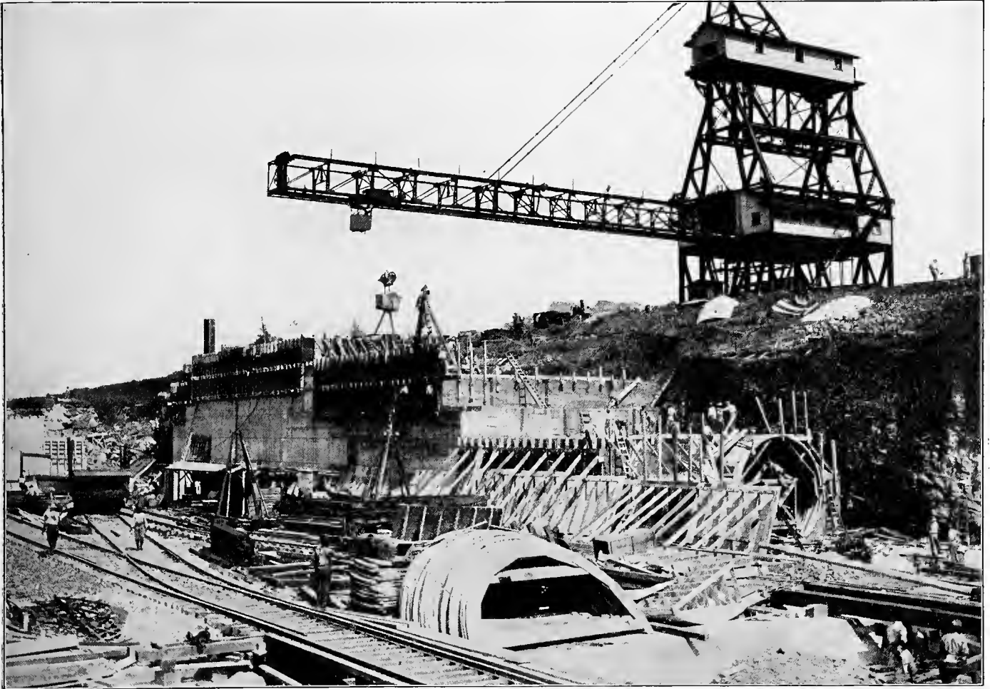
TRAVELING CRANE HANDLING CONCRETE IN LOCK-BUILDING
